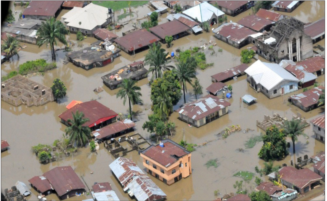
Plate 2: Houses destroyed by flood in Ganaja
