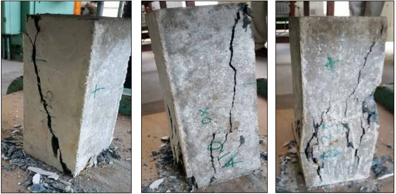
Figure 19. Failure mode and pattern of axial compression of (a) CTR, concrete, (b) NonC, and (c) N treated NSFRC prisms
